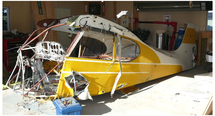
My new prize. The boot cowl and firewall have been removed exposing the damage to the forward fuselage
