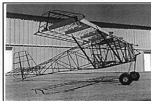
The Buttercup under construction.
