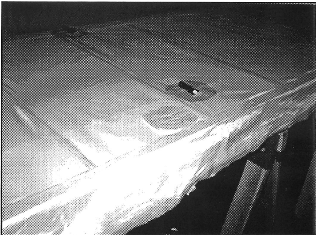
Fabric which has been glued to the lower side of the wing. Note areas around the strut brackets, covered with cement and ready for re-inforcement patches.
